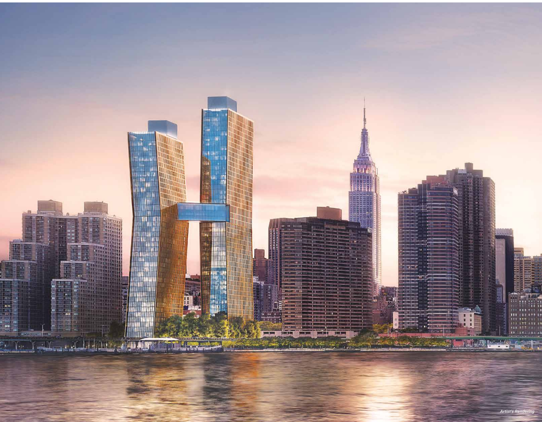
American Copper Buildings / New York
